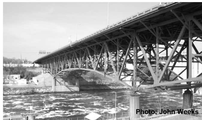
Fig. 1: A view of the I-35W bridge looking northeast
